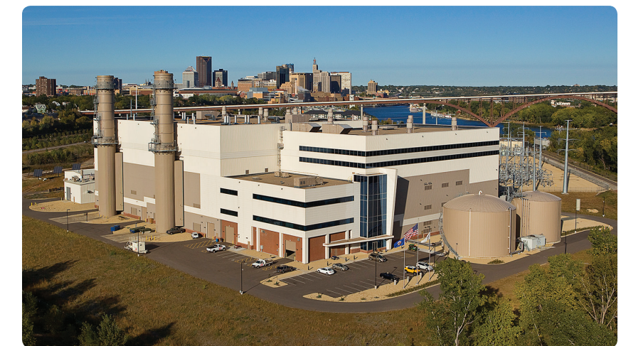
Converted for natural gas production, the Xcel Energy High Bridge Generating System in Saint Paul came on line in May 2008.
