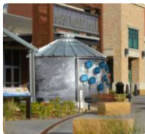
Maplewood Mall 55 rain gardens, 6,733 square feet of permeable pavers, 375 trees, and one decorative 5,700-gallon cistern built to catch stormwater greet visitors. Together, they help intercept 20 million gallons of runoff per year before it reaches nearby Kohlman Lake.
